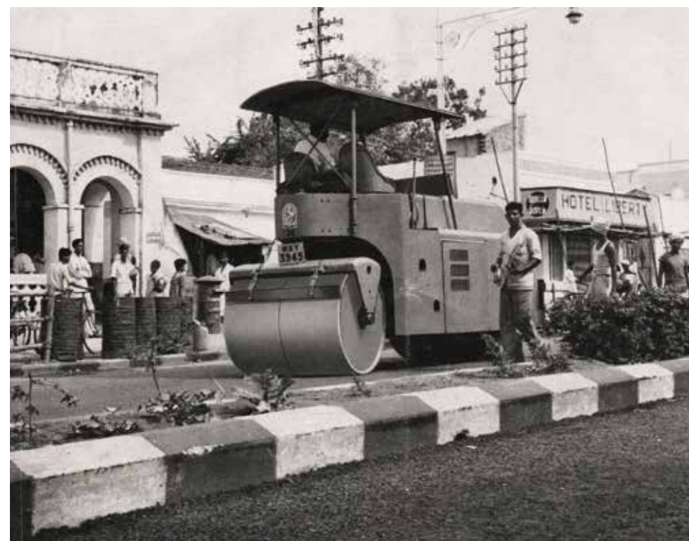
Another later design of Aveling-Barford roller – the TR tandem – is seen at work in Madras, now Chennai.
