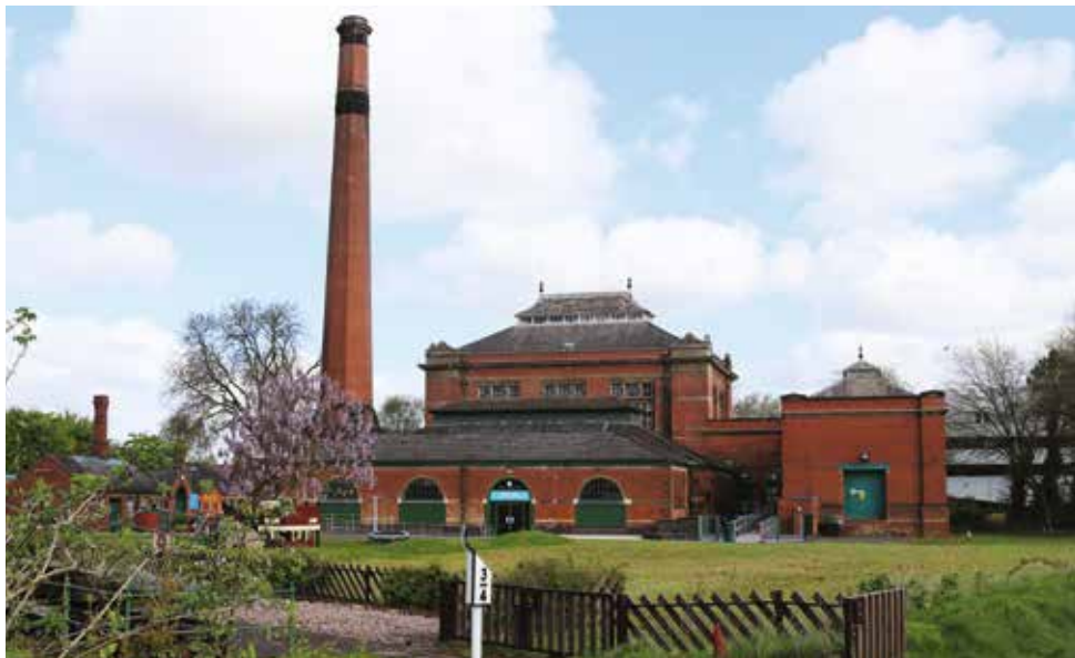
A view of Abbey Pumping Station from the riverside path.
