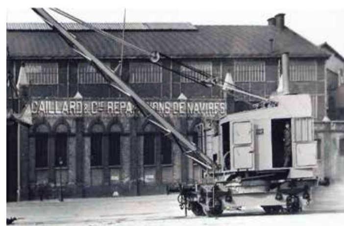
One of Caillard's steam cranes. Author's collection
